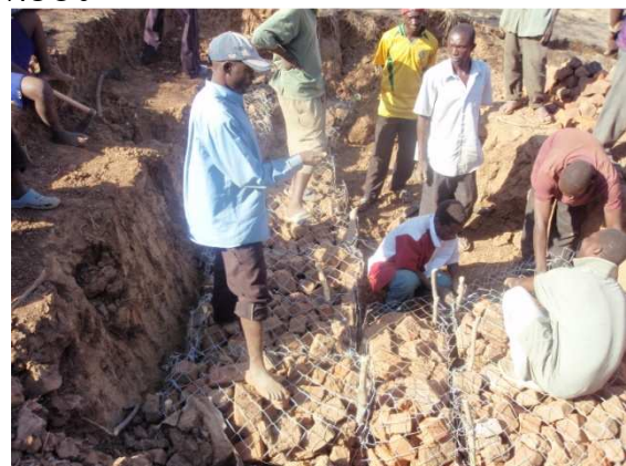
Figure 7: Mbire community members reclaiming a gully.
